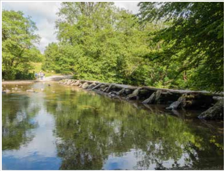
TARR STEPS is a clapper bridge over the River Barle. Its age is unknown, however several theories claim that Tarr Steps dates from the Bronze Age but others date them from around 1400 AD.
